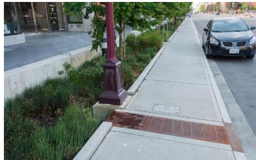
Road side SUDS planting
